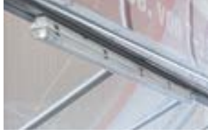
Interior lighting Weatherproof design with 58 watt lights.
